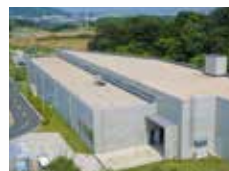
Energy Center (Facility for combined energy and water treatment)
